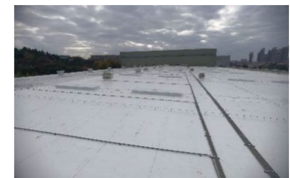
The renovated warehouse
