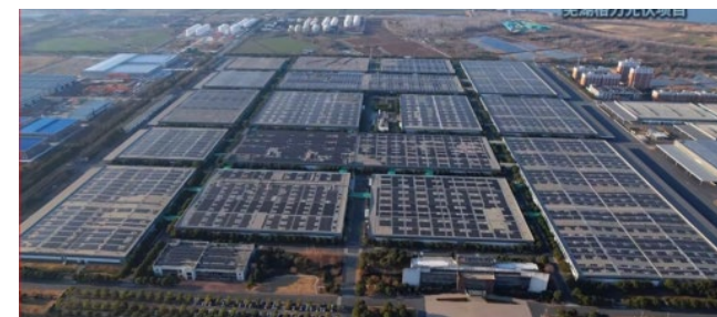
GREE Wuhu PV Project
